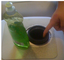
Insert drain lip into seal
