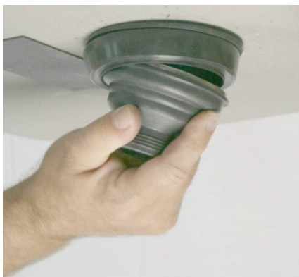
Insert drain lip into seal
